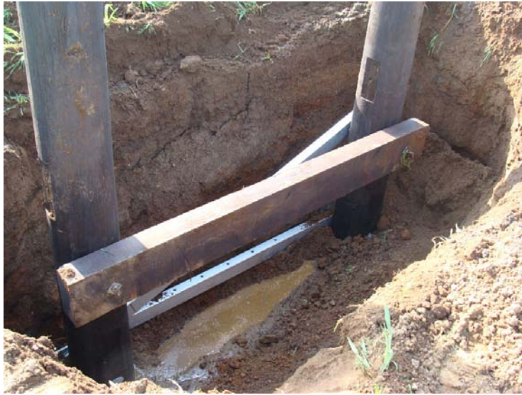
▲ Construction of Section Angle Support Pole
