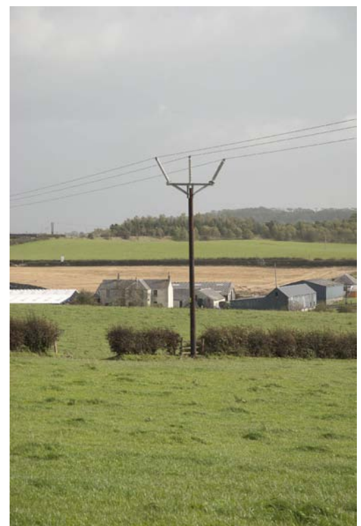
Trident 43-50 Intermediate Support Pole
