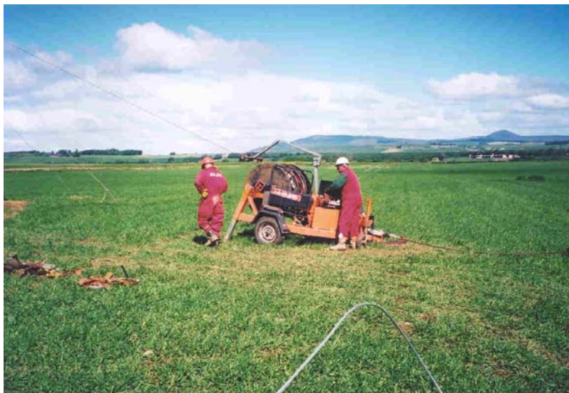
▲ Winch for Stringing Wood Pole
