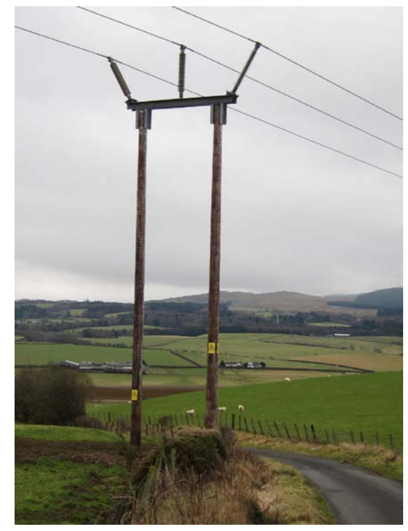
Long span intermediate 'H' pole
