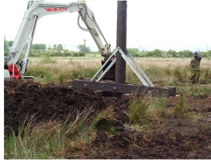
▲ Construction for Intermediate Support Pole in Soft/Boggy Ground Conditions
